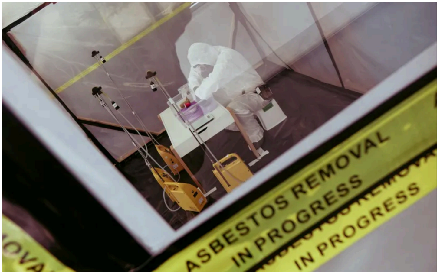
Asbestos removal is carried out. Kim Baker Wilson / RNZ
