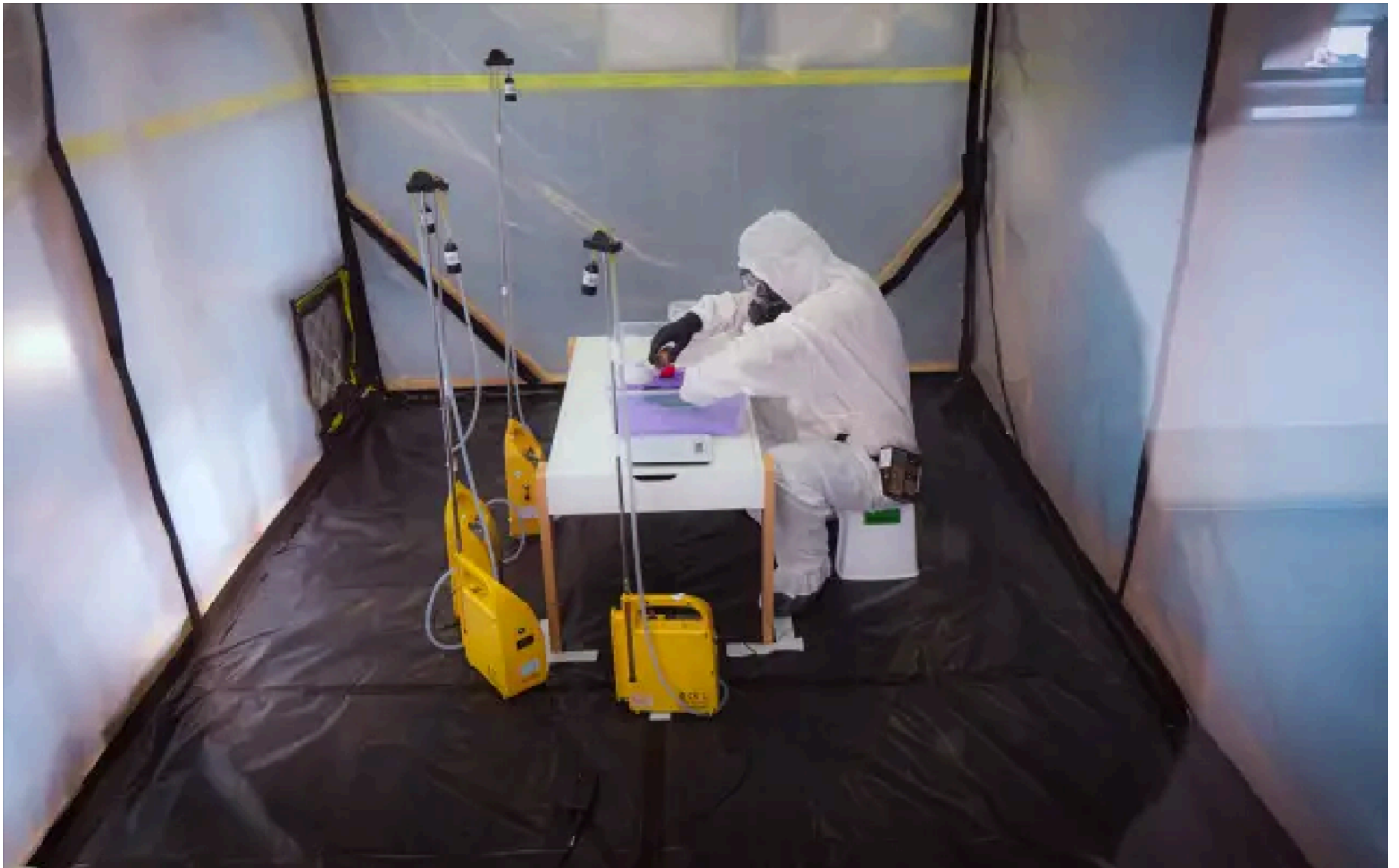
Asbestos testing is carried out. Kim Baker Wilson / RNZ
